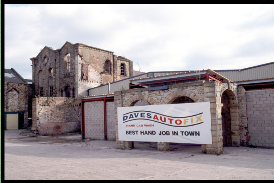
Fire damage to historic mill
